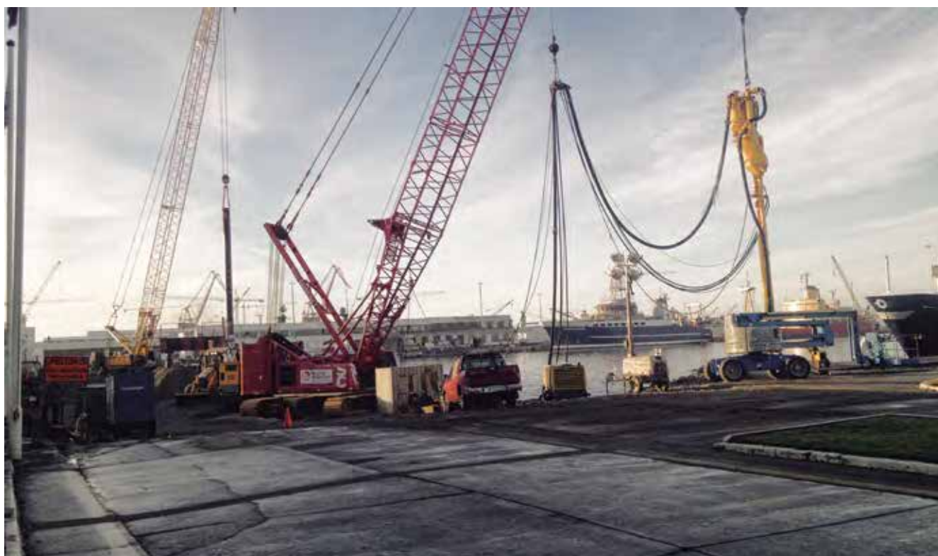
Columnas de Grava Off Shore, Puerto Asmar Talcahuano, Bío Bío - Chile
