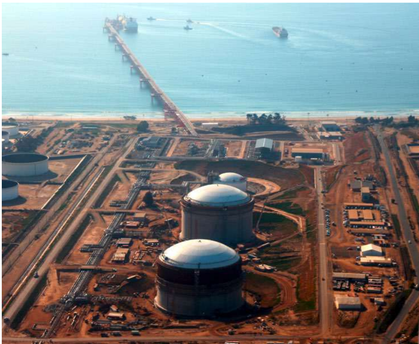
Terminal GNL Quintero
