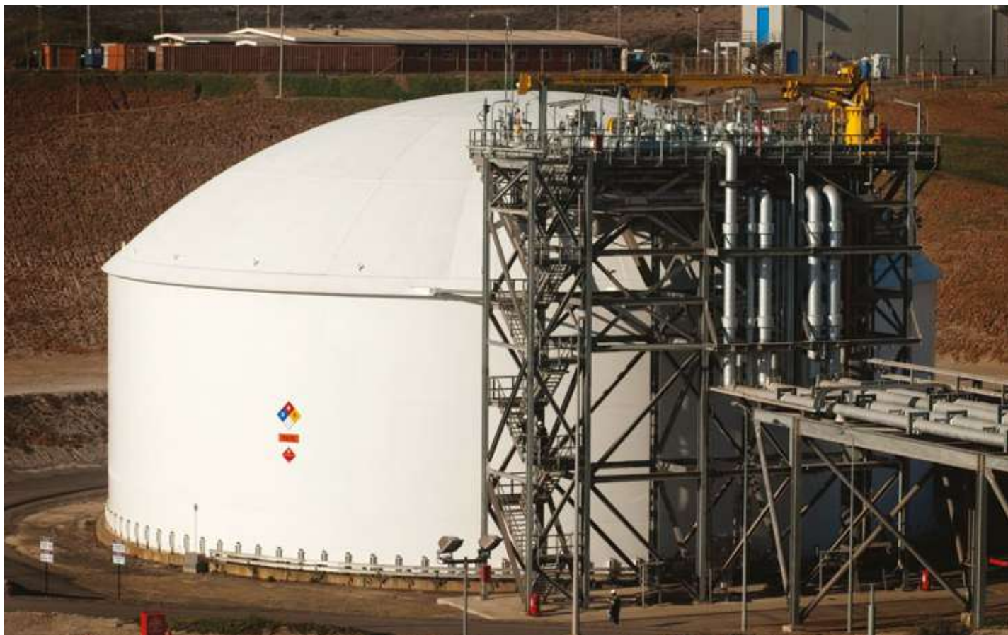
Terminal GNL Quintero
