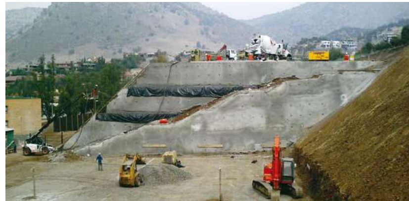
Soil Nailing, Colegio Everest
