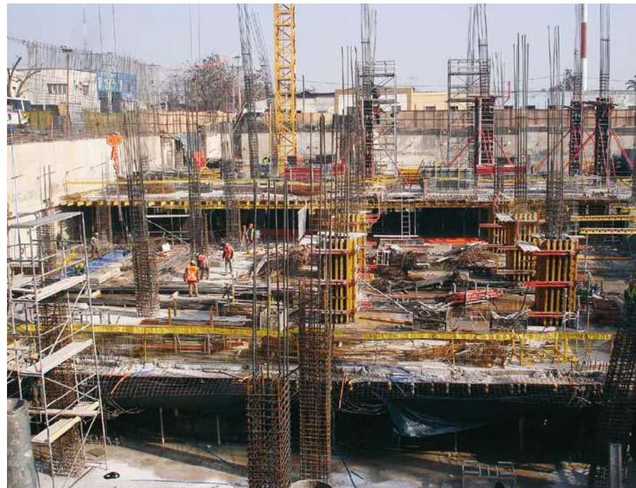
Losa Postensada Mall Plaza Alameda
