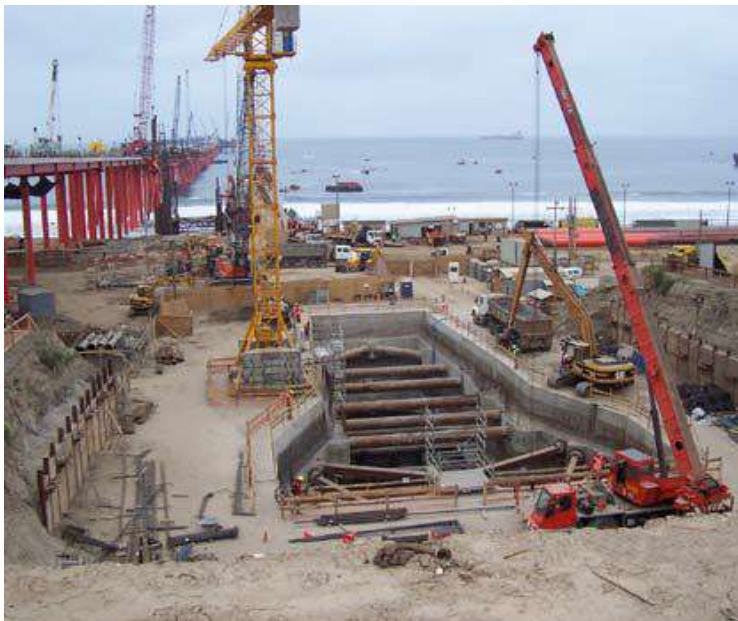
Muro Pantalla Sea Water Intake, GNL Quintero
