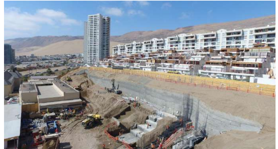
Soil Nailing sede Instituto Inacap, Iquique
