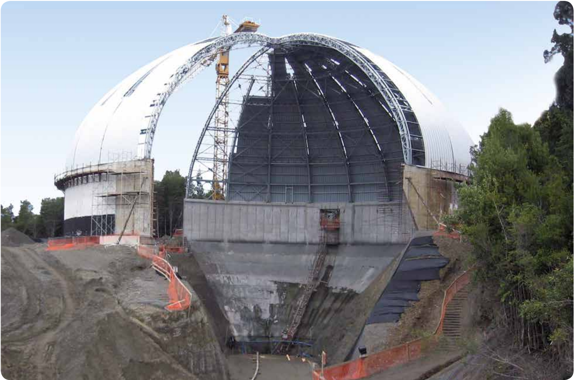
Domo puerto industrial Calbuco, Lafarge - Puerto Montt
