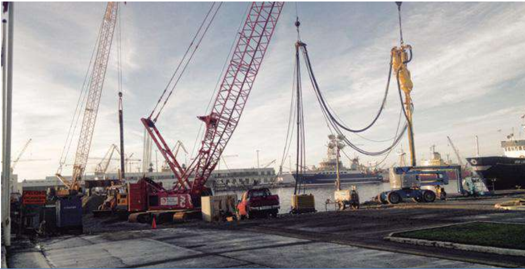
Columnas de Grava Off Shore, Puerto Asmar Talcahuano, Bío Bío - Chile
